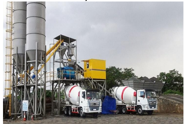
Gambar 2. Fasilitas Ready mix
